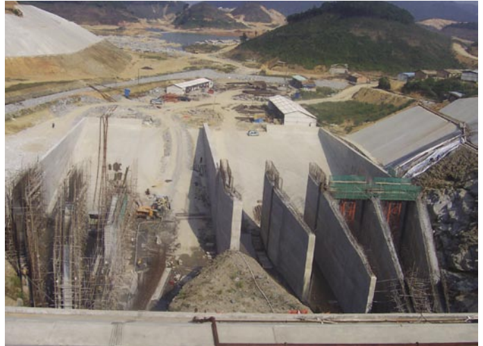
Construction of the upper reservoir of the hydro power plant Bailianhe.
